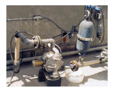
pressure driving the pump motor, the pump just stops or *stalls* with no pressure relief required and no damage to the pump.
